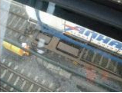
Photograph 10: Crane operator's view of the loading operation
